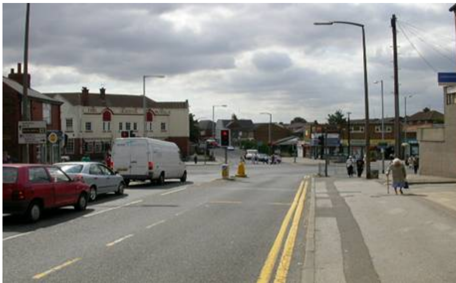
Figure 4.6 - Junction of High Street/Tickhill Road/Grange Lane/Muglet Lane
